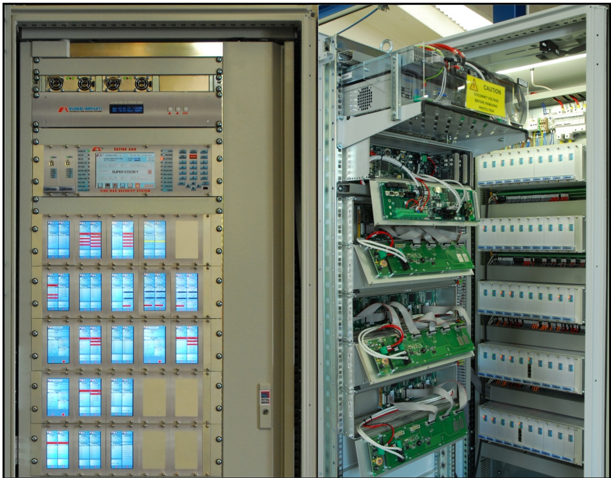
EXFIRE360 fire&gas control panel (views from outside and inside)
